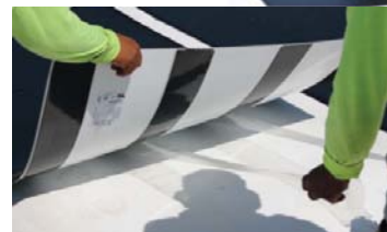
Peel & Stick Modules to TPO
