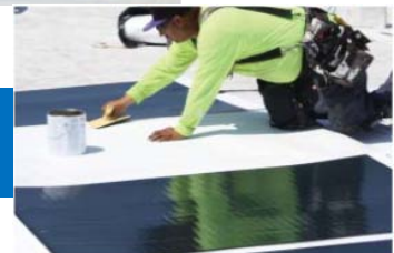
Peel & Stick Modules to TPO
