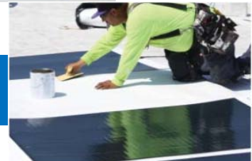
Peel & Stick Modules to TPO
