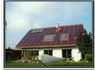
Residential Rooftop PV system
