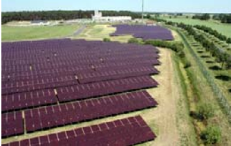
Capacity: 3.7MW Type: Ground Mounted Location: Schonewalde, Germany
