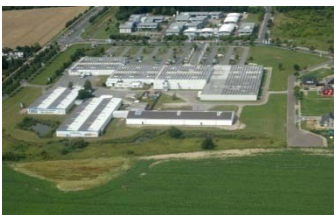
Capacity: 485KW Type: Rooftop Location: Magdeburg Germany
